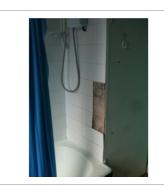
Damaged tiles. Several tiles have broken off of the wall. Could create a sharp surface - hazard. Replace tiles. 3
