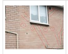
External wall has a cavities and cracks, and repairing it is recommended. Hire a competent person to do so. 3
